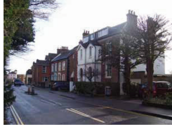
Fig 146 Churchfields Road Villas
