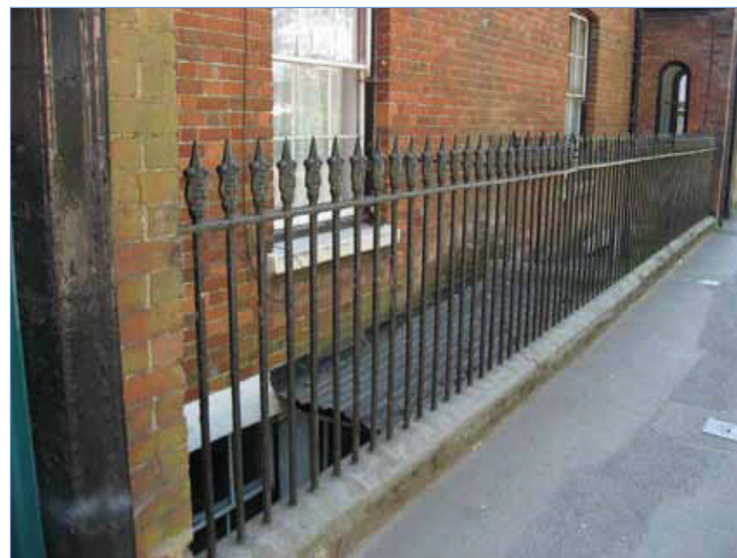
Fig 84 Cast iron railings
