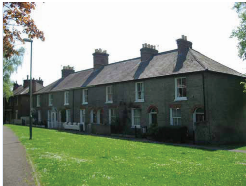
Fig 51 East of Greencroft Street
