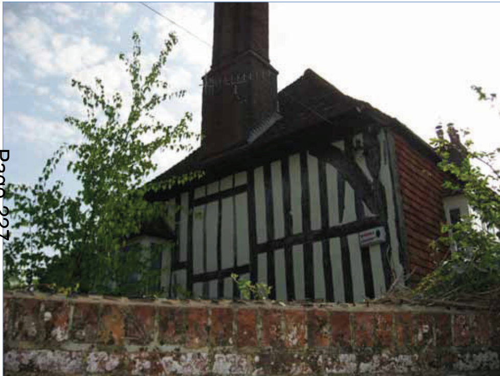
Fig 102 Timber framing, Harnham Road
