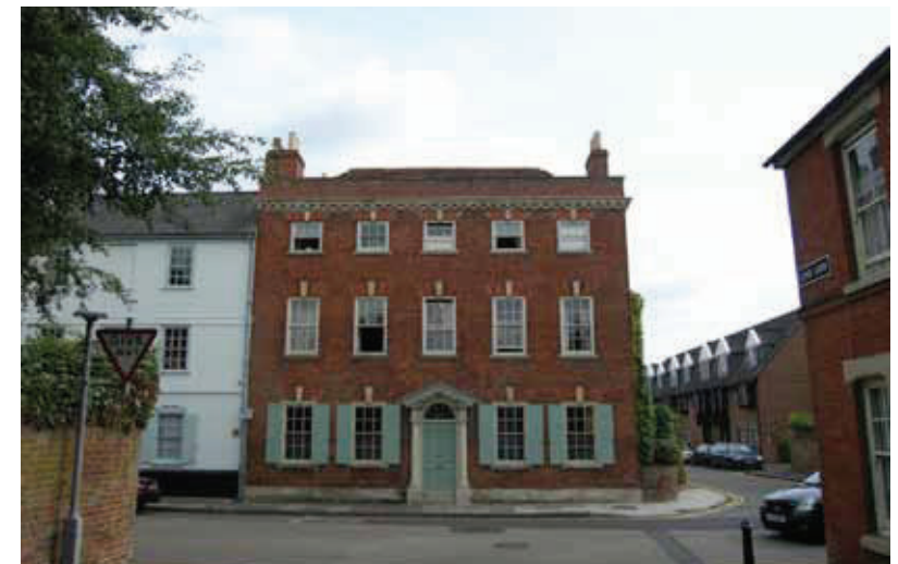
Fig 124 larger scale Georgian house, Vale House, No. 44 St Ann Street
