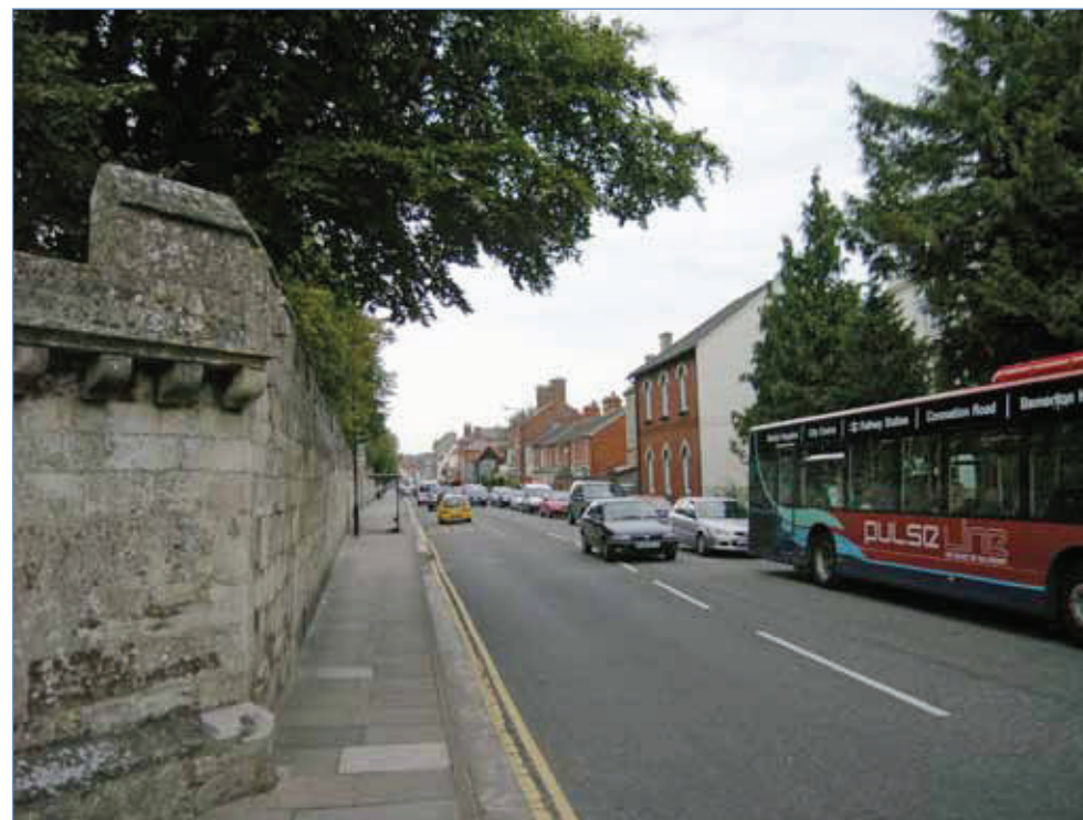
Fig 70 View of Close wall from Exeter Street
